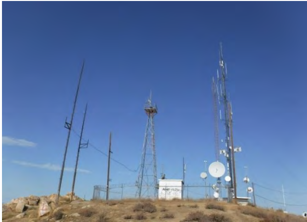
Box Springs Communications Site
