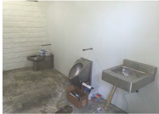
Park Restroom Renovations
