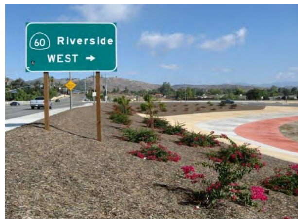
SR-60 / Nason Street Overcrossing Bridge (Landscape Establishment)
