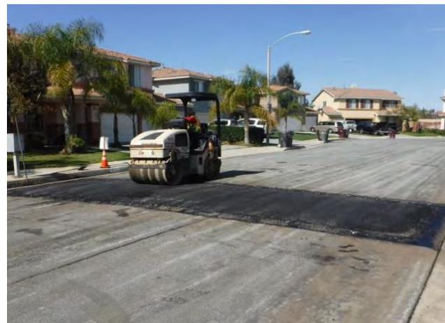
Residential Traffic Management Program (Speed Hump Program)
