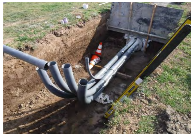
Feeder Line Trenching
