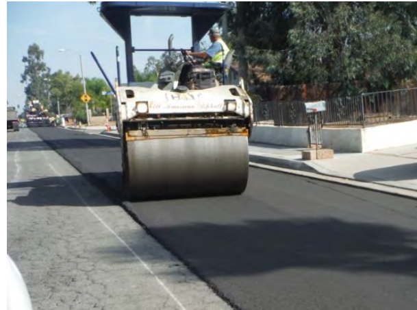
Citywide Annual Pavement Resurfacing Program
