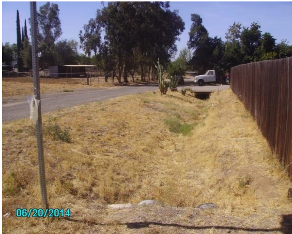
Photo 3: Existing drainage along west side of Carrie Lane (looking south).
