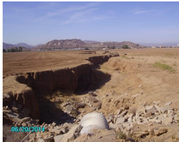
Photo 8: Culverts outlet downstream of Ironwood Ave. (looking south).
