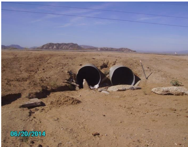
Photo 7: Culvert outlet downstream of Ironwood Ave. (looking north).
