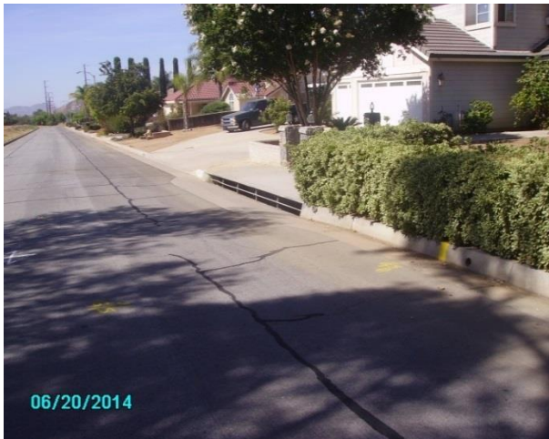
Photo 5: Storm drain on west side of Pettit Street (looking south).
