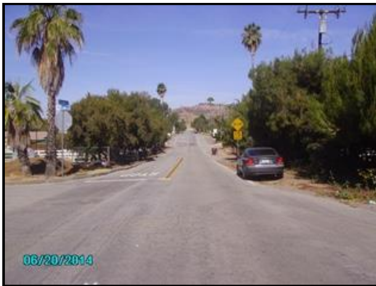
Photograph D: Kalmia Avenue near Carrie Lane (facing westward)
