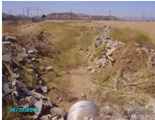
Photo 6: Culvert within incised channel downstream of Pettit Street outlet (looking south).
