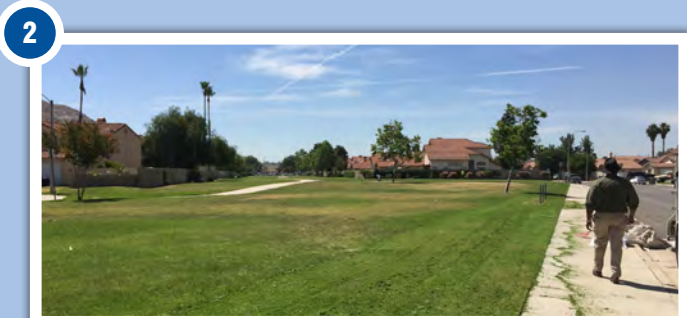
2 Psomas will validate the adequacy of path radii in this segment of the alignment. A minimum design speed of 20 mph will be used as the parameter to guide this assessment.
