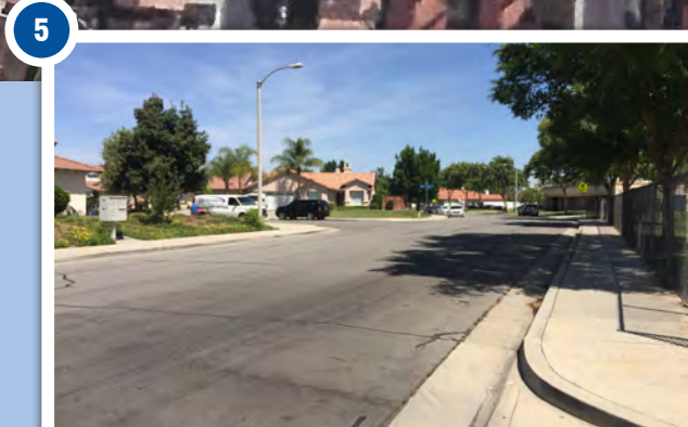
5 Instead of having bike routes on both sides of Via Pamplona, Psomas proposes a two-way buffered bike lane on the west side instead to avoid conflicts with curb-side parkings, loading zone and parking lot ingress/egress access. Northbound to eastbound cyclists directly accessing schools can still share the road with motor vehicles. All of which promotes safety and enhances connectivity to the new path.
