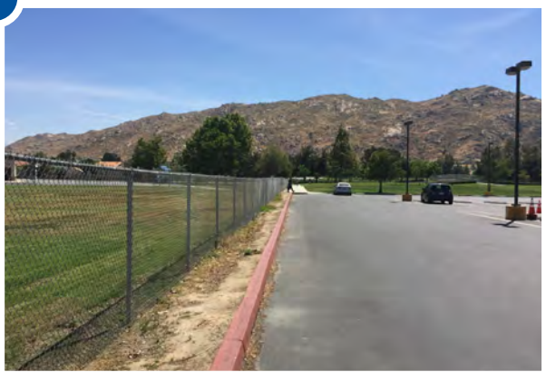
3 View of connection to the existing PCC walkway located further east in the park. Depending on final cross-section configuration selected, additional PCC may need to be constructed along with DG path for pedestrians.
