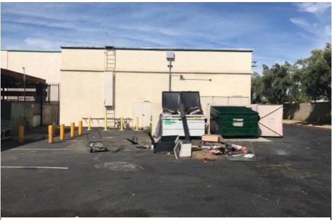
Existing trash enclosure-Northwesterly of property
