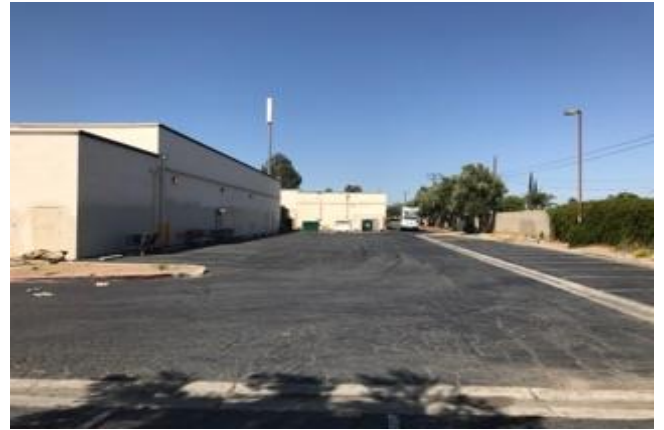
Existing conditions (north of property)-looking west
