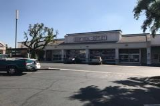
Existing Front entrance-West of property
