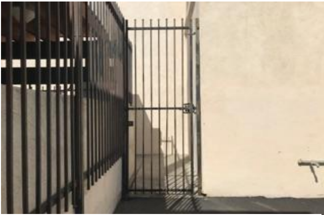
Existing metal gate-Northwesterly of property
