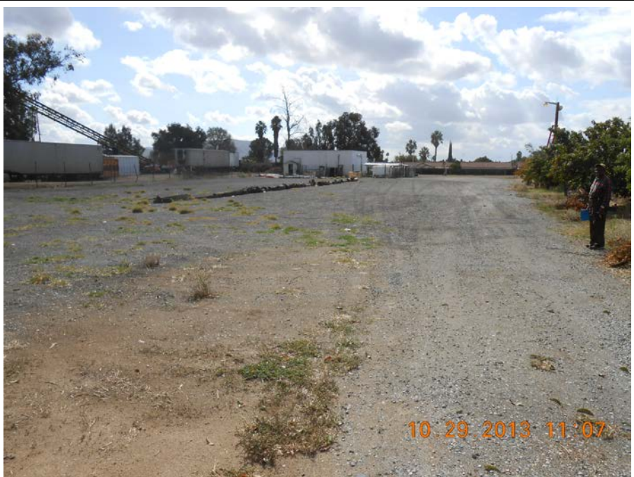
Photograph 3: Southerly view of the central portion of the subject property taken from the southwest corner of the existing residence.
