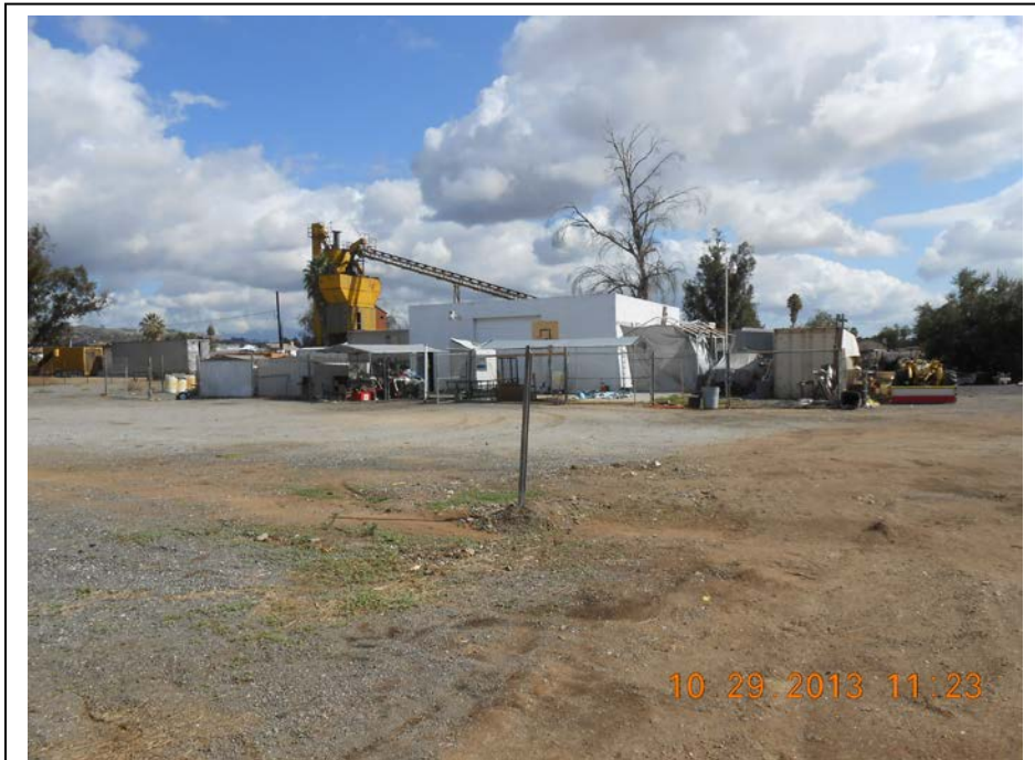
Photograph 9: Easterly view of the storage garage area in the southern portion of the site, taken from the parcel to the west. Orange tower is offsite.
