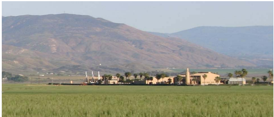
San Diego Gas & Electric Natural Gas Compression Station
