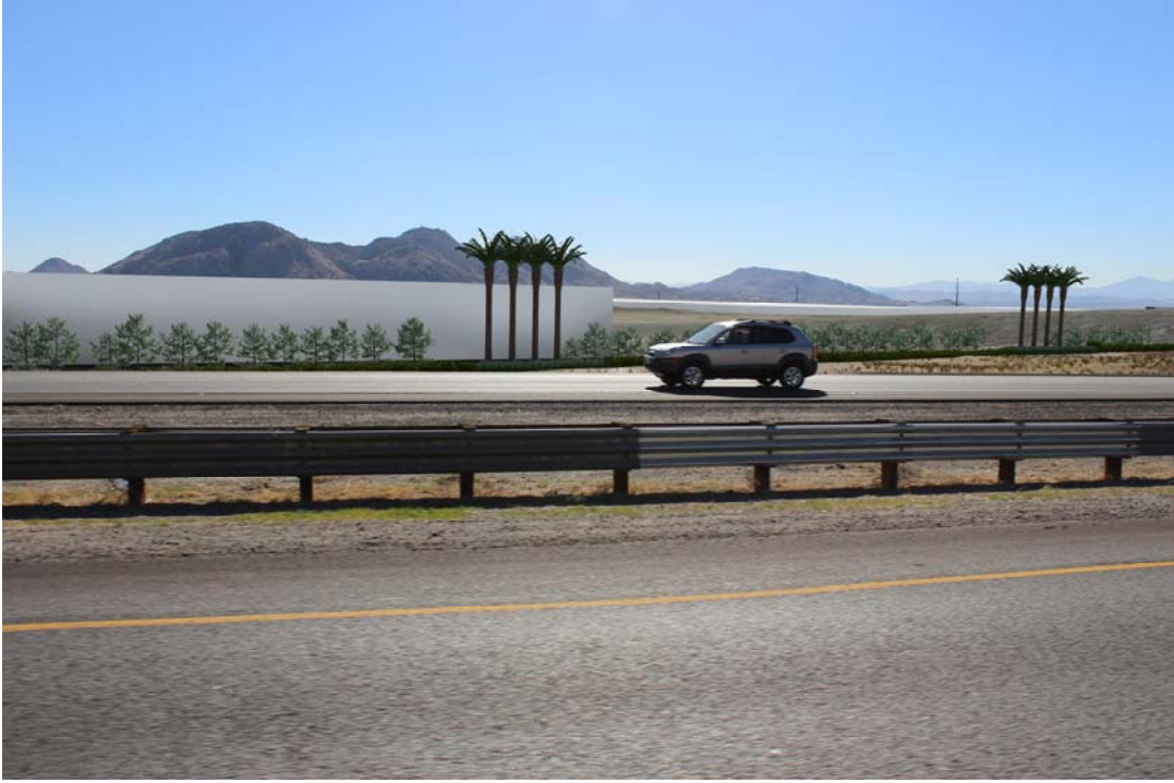
60 Freeway View 8 at Installation
