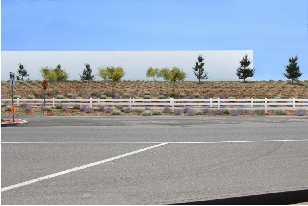
Redlands Blvd. View 3 at Installation
