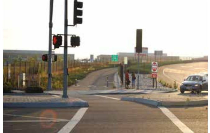
Class 1 bicycle path at-grade crossing - San Diego, CA
