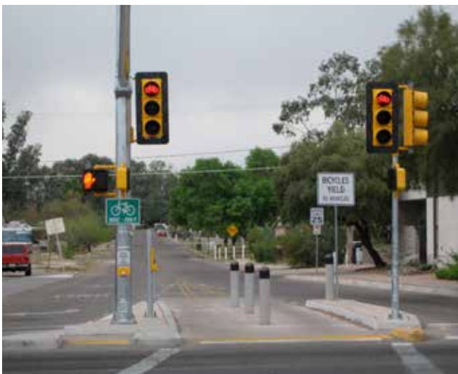
Bicycle signals - Tucson, AZ
