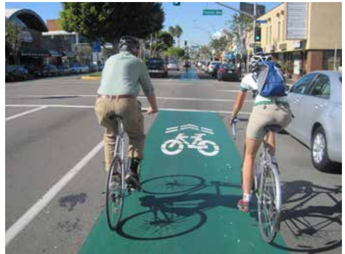
Green striped lane with shared lane markings - Long Beach, CA)
