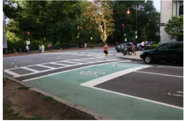
7B) Bike boxes are advanced stop bars for cyclists that provides them room to cue up in front of other vehicles waiting at a red light. While this treatment is still considered experimental, it is thought to increase cyclists' visibility, and therefore safety - Cambridge, MA
