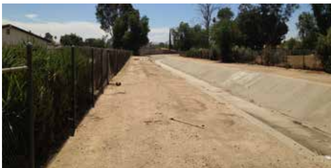
Typical flood control channel
