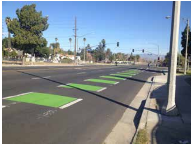
Green lane and merge zone - Riverside, CA
