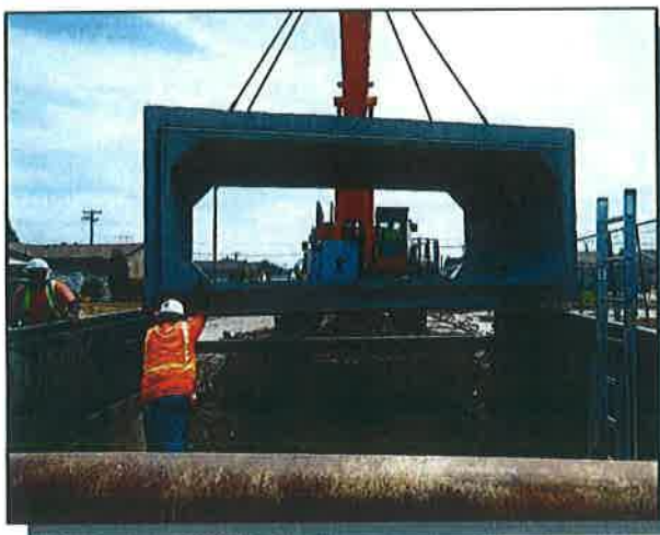
Reinforced Concrete Box
