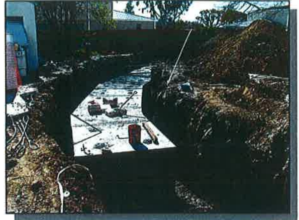
Downstream portion of 6.0'Wx3.5'H Reinforced Concrete Box
