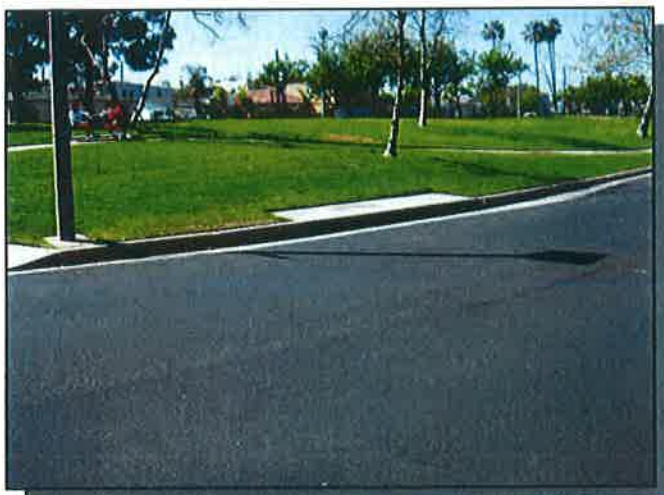
Electric Avenue (north) - Catch Basin Inlet
