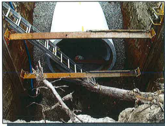
Electric Avenue Storm Drain
