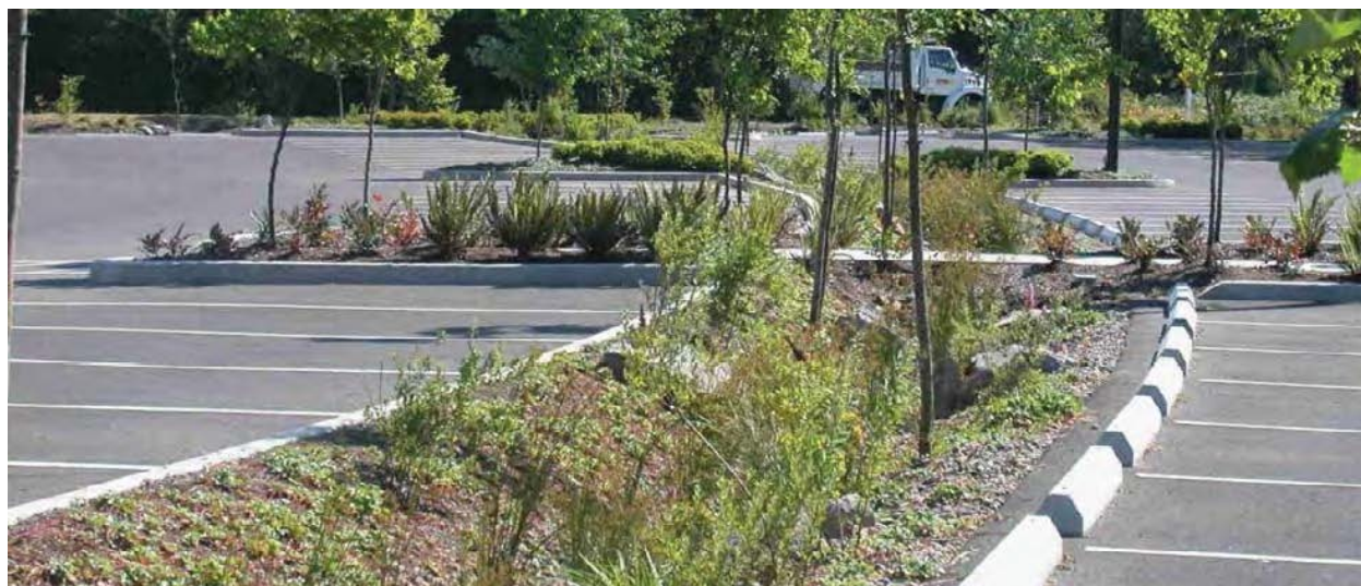
Figure 5-7 Example of Biodetention Facility
