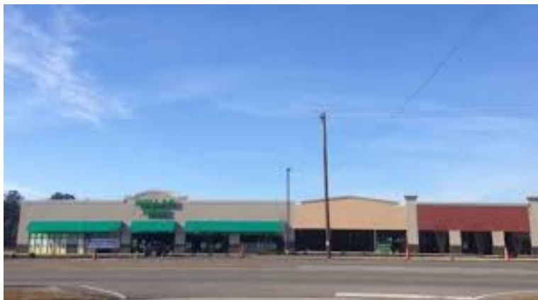
Figure 5-19 Example of Inappropriate Characteristics for Retail
