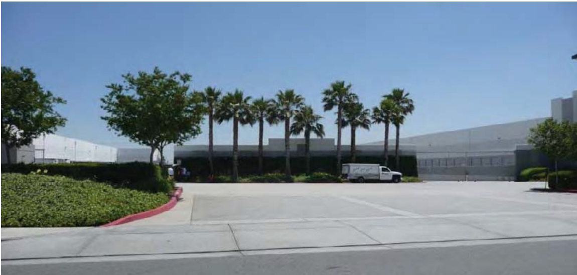
Figure 5-25 Example of Appropriate Ground Mounted Equipment Screening
