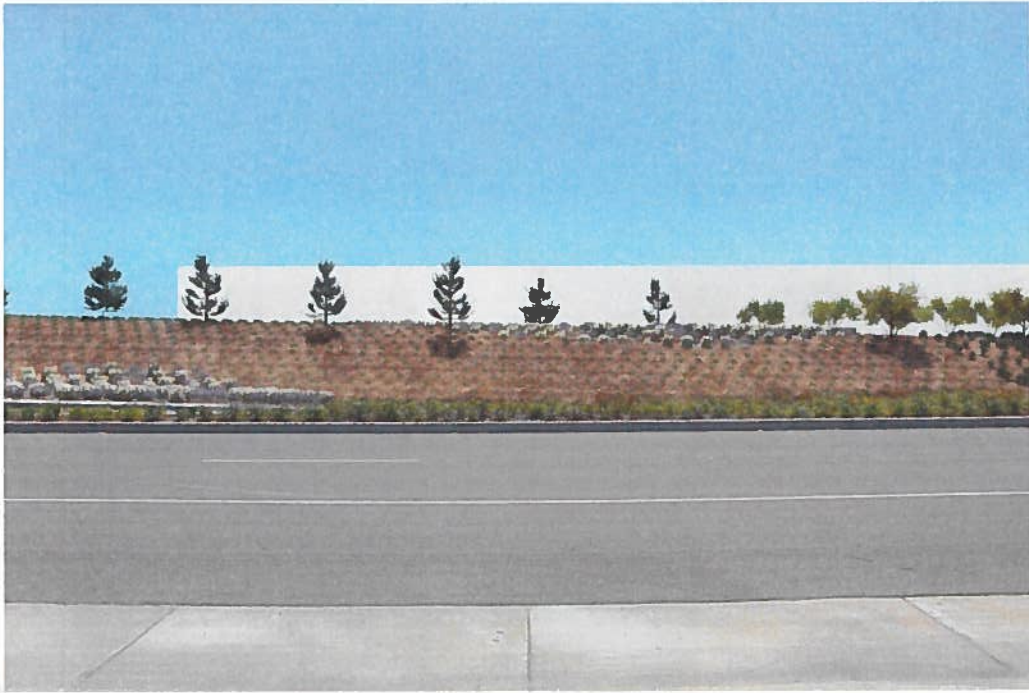
Redlands Blvd. View 1 at Installation
